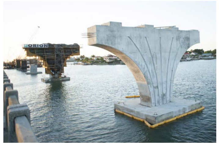
Figure 3: Column/Pier Construction (Source: www.newbaywaybridge.com)
