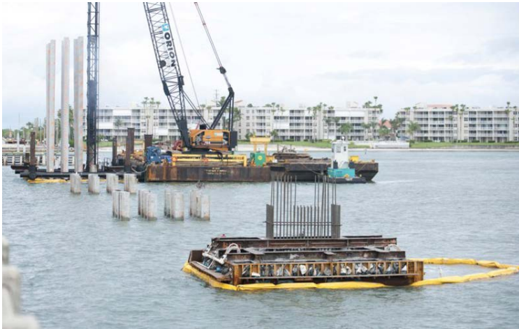
Figure 2: Pile Driving and Footing Formwork (Source: www.newbaywaybridge.com)
