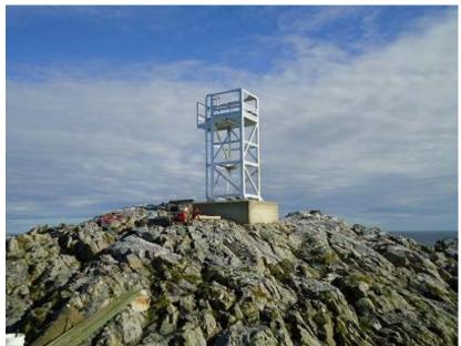
Figure 4: Implemented Gravity Based Tower at Gull Rock (Source: Canadian Coast Guard)
