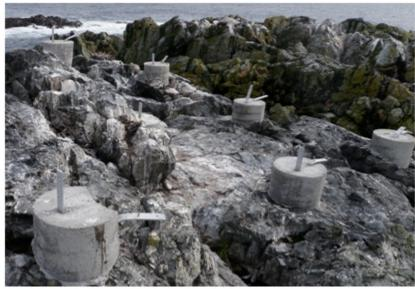
Figure 5: Horizontal Failure of Helicopter Pad Supports (Source: Canadian Coast Guard)
