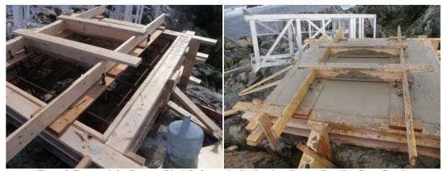
Figure 3: Formwork for Concrete Block Before and After Pouring (Source: Canadian Coast Guard)
