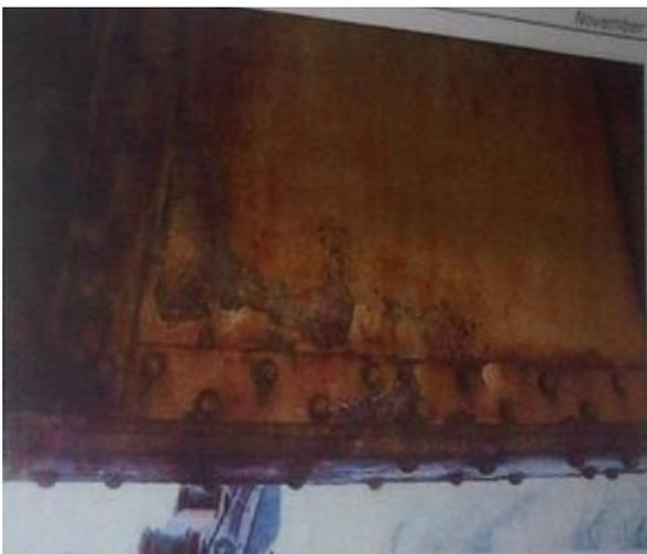
**Figure 7: Failure of structural steel coating system**
