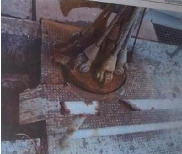
**Figure 9: Failure of steel platform**
