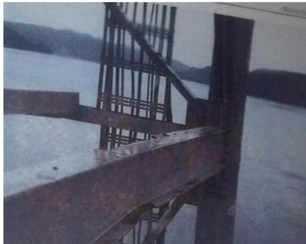
**Figure 8: Deformation due to accident damage**
