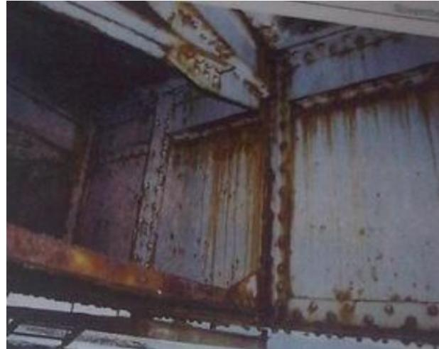
**Figure 10: Typical severe corrosion at main girder**
