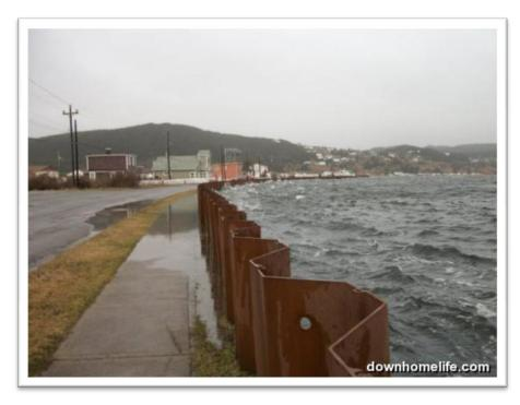
Figure 6: Extremely high tides against the Placentia sheet pile Flood wall (Source: <a href="www.downhomelife.com">www.downhomelife.com</a>).
