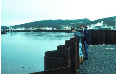
Figure 3: Sheet pile floodwall along the backside of Placentia (Source: www.heritage.nf.ca)
