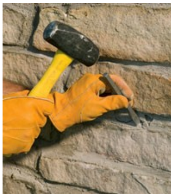
Figure 2: Chipping out damaged mortar
