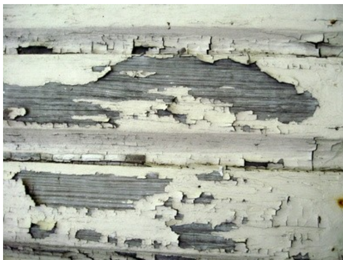
Figure 3: Discolouring from oxidization
