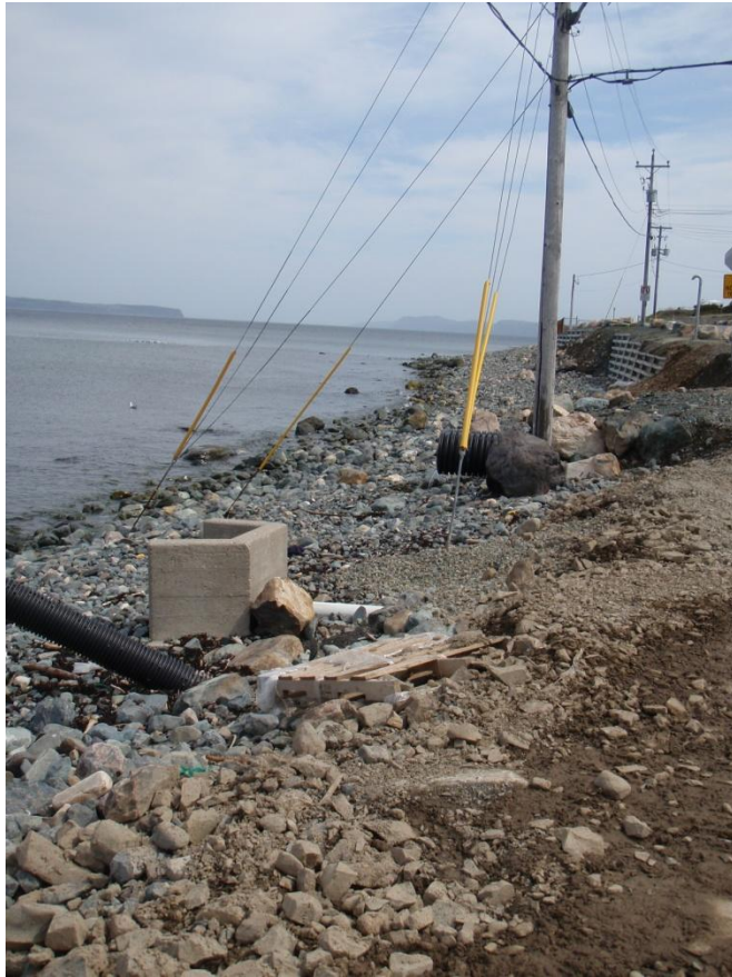
Figure 5: Exposed infrastructure along Goodland Road (Source: Personal Photo)
