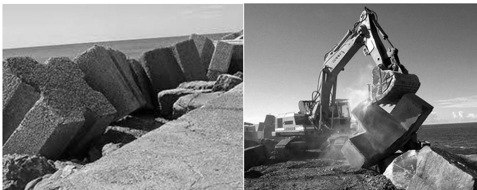
Figure 6 An Example of Antifer Cubes (Left) and Hanbar units (Right)
