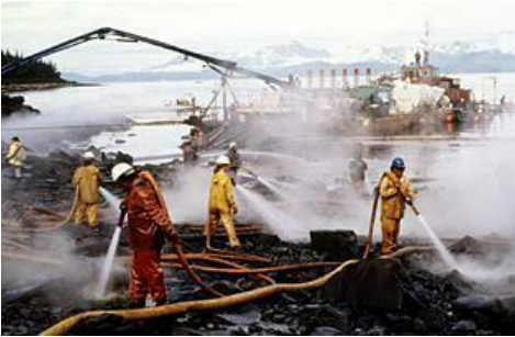
Figure 2.2: High Pressure Water
