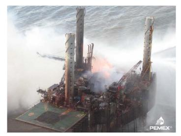
Figure 4: Collapse of the Usumacinta's Derrick and Heavy Damage Caused by the Second Fire
