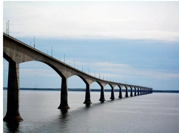
Figure 2 Confederation Bridge Section showing concrete marine piers [3]
