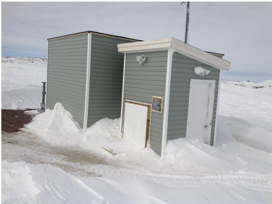
Figure 1. The Potable Drinking Water Unit, Black Tickle, April, 2013.
