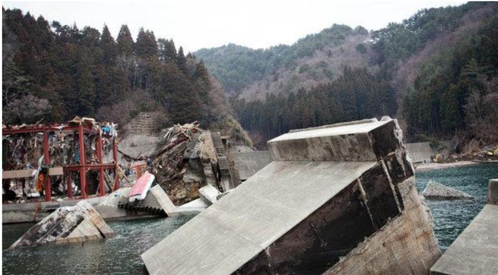
Figure 7: A section of the destroyed Kamaishi breakwater
