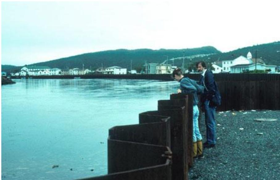
**Figure 3: Sheet pile floodwall along the backside of Placentia**
