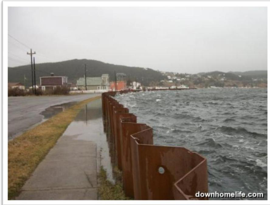
**Figure 6: Extremely high tides against the Placentia sheet pile Flood wall (Source: [www.downhomelife.com](http://www.downhomelife.com)).**
