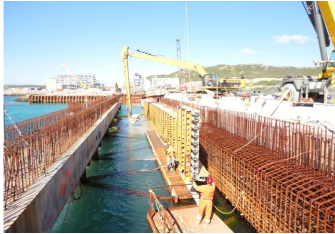
Figure 3: Placing Scour Protection. Photo Credited to PMJV.
