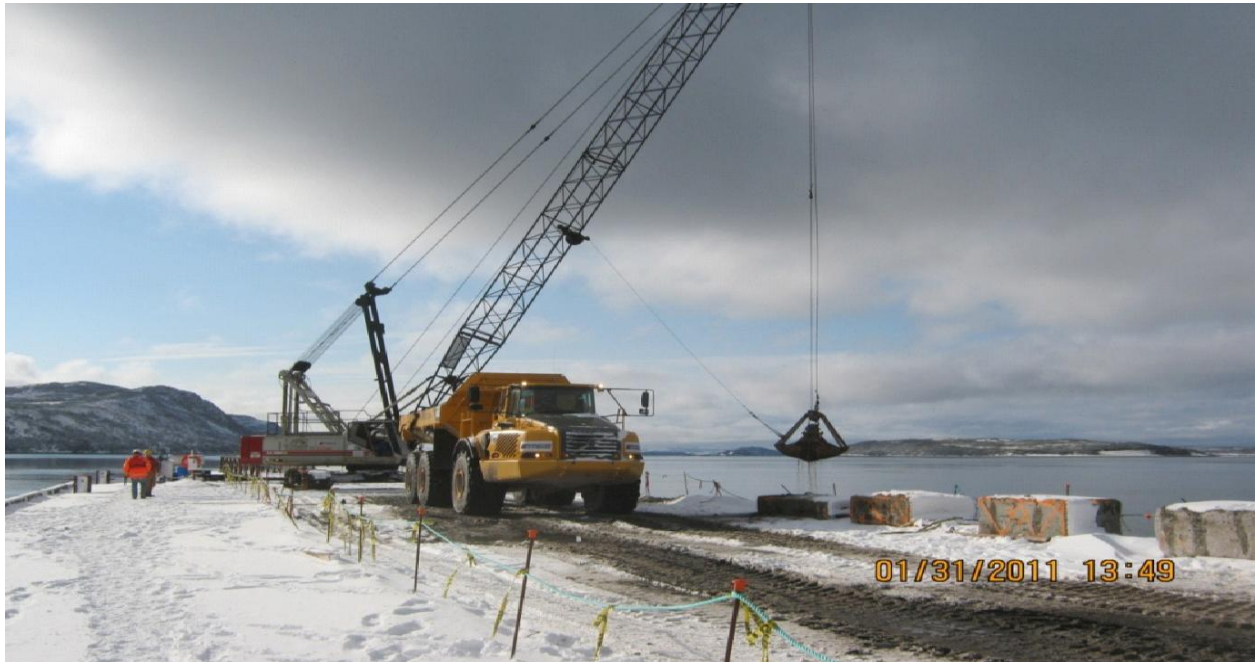
Figure 2: Dredging. Photo credited to PMJV.
