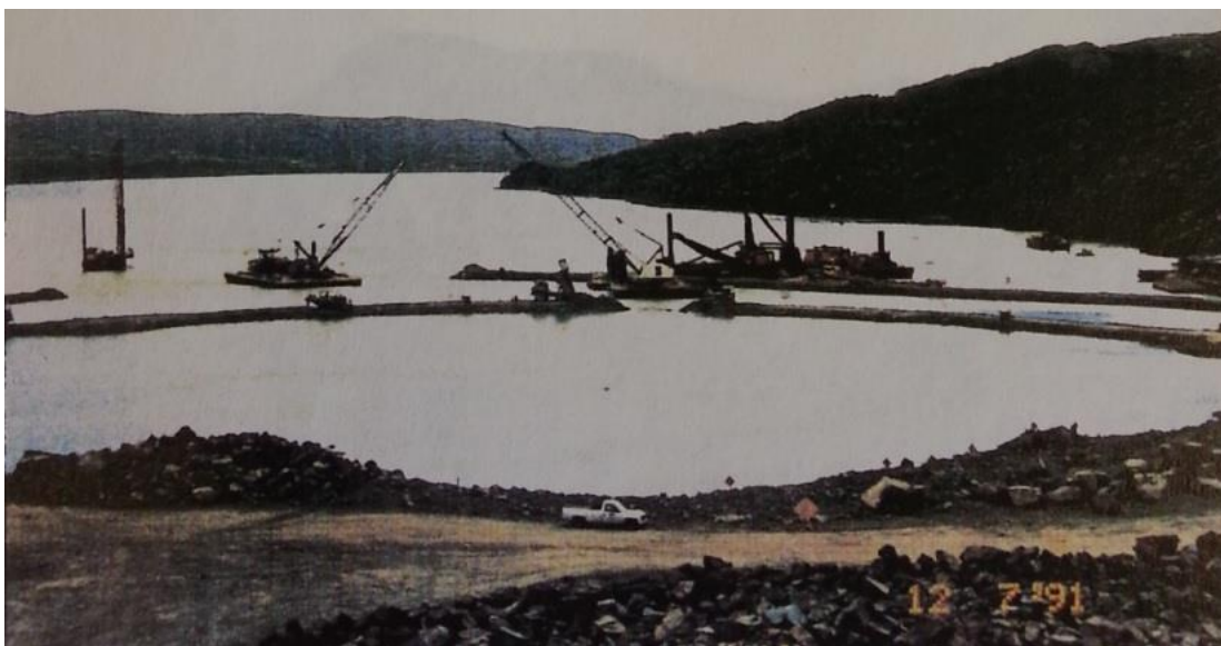
Figure 5 – Hibernia Berm Construction
