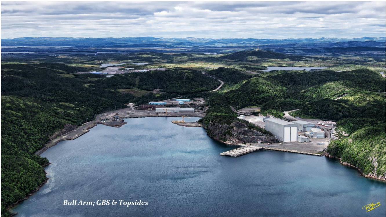
Figure 2 – Bull Arm Fabrication Site
