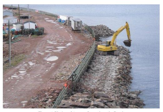
Figure 6: Placing of Armour Stone along the Beach
