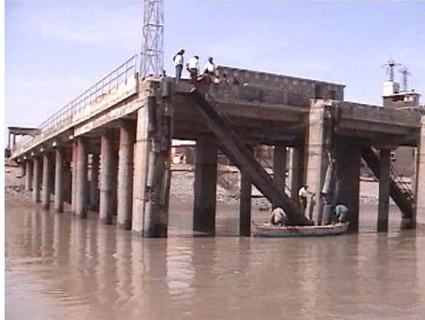
Figure 4 – Wharf Supported by Steel Piles
