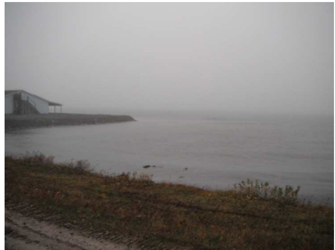
Figure 6 – Bear Cove Project Completion
