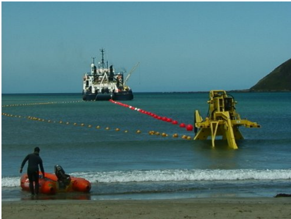
Figure 3b: Cable Ship with Sea Plough and Cable Buoys
