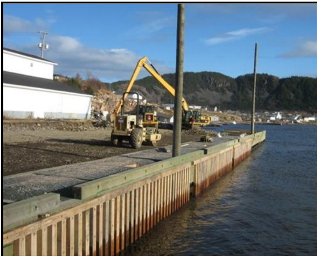
Figure 6: Marginal Wharf Construction (Source: CBCL Limited Consulting Engineers)
