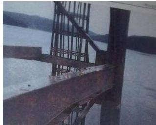
Figure 8: Deformation due to accident damage (Source: Delcan Inspection Report, 2011)
