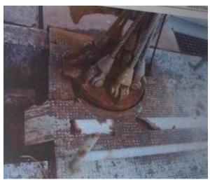
Figure 9: Failure of steel platform Source: (Delcan Inspection Report, 2011)
