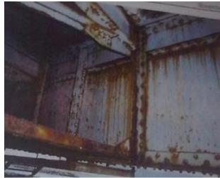
Figure 10: Typical severe corrosion at main girder Source: (Delcan Inspection Report, 2011)
