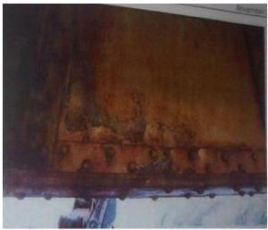
Figure 7: Failure of structural steel coating system (Source: Delcan Inspection Report, 2011)
