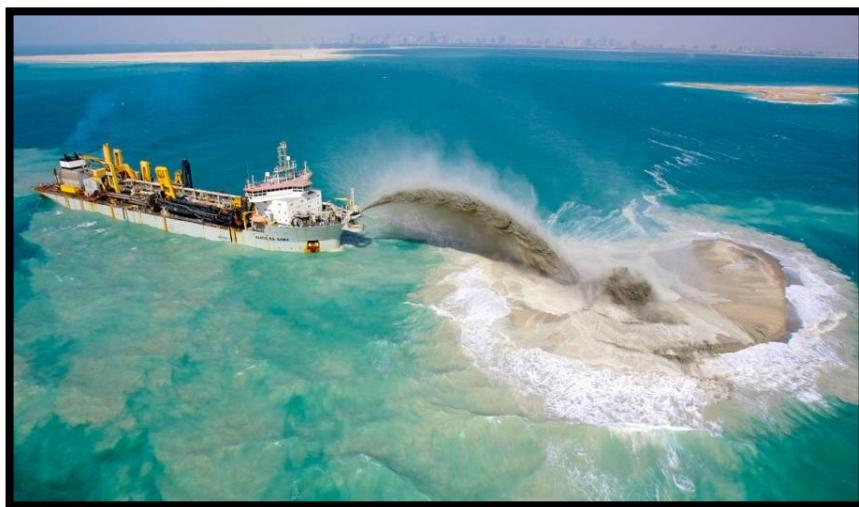
Figure 4: The process of rainbowing sand to create Palm Jumeriah's fronds
